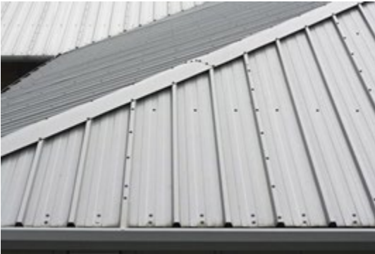
Exposed Fastener Metal Roof
